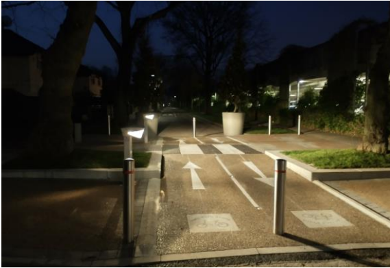
Low level lighting can be used in areas where traditional street lights are not suitable.
