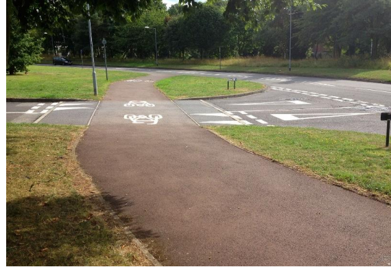
Cycle priority can be provided over side roads, with a set back on busier or faster roads.
