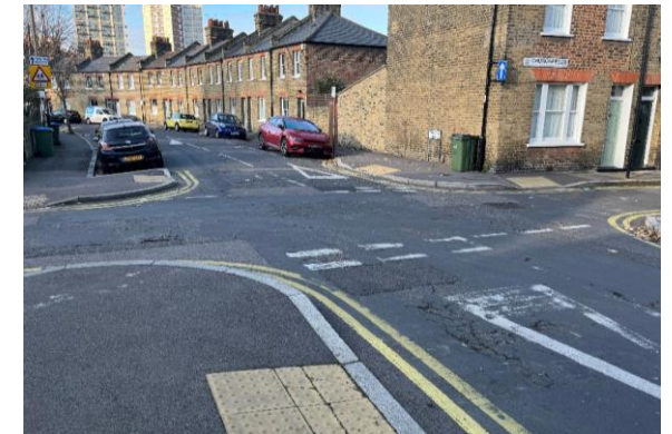
Tightening the junction radius can have the effect of slowing turning traffic and encourage drivers to give way to pedestrians crossing side roads.
