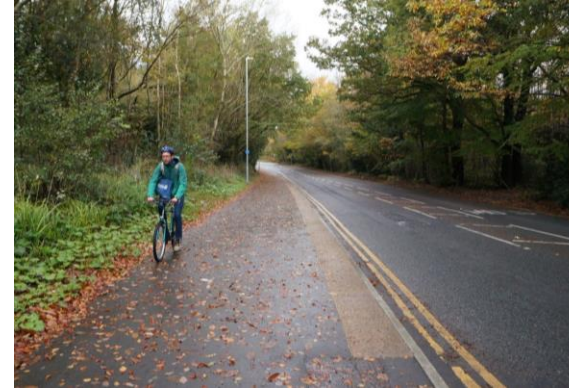
Wide shared use paths can be suitable where footfall is low alongside main roads.
